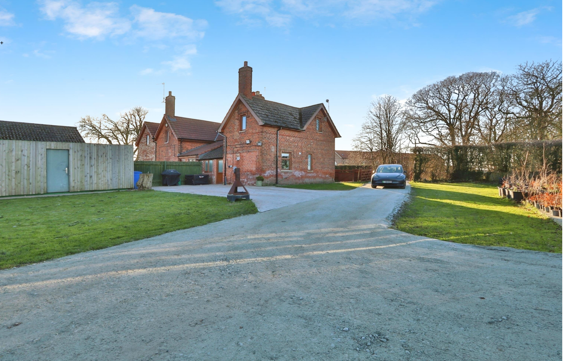
2 Enholmes Farm Cottage, Enholmes Lane, Patrington, HU12 0PR
