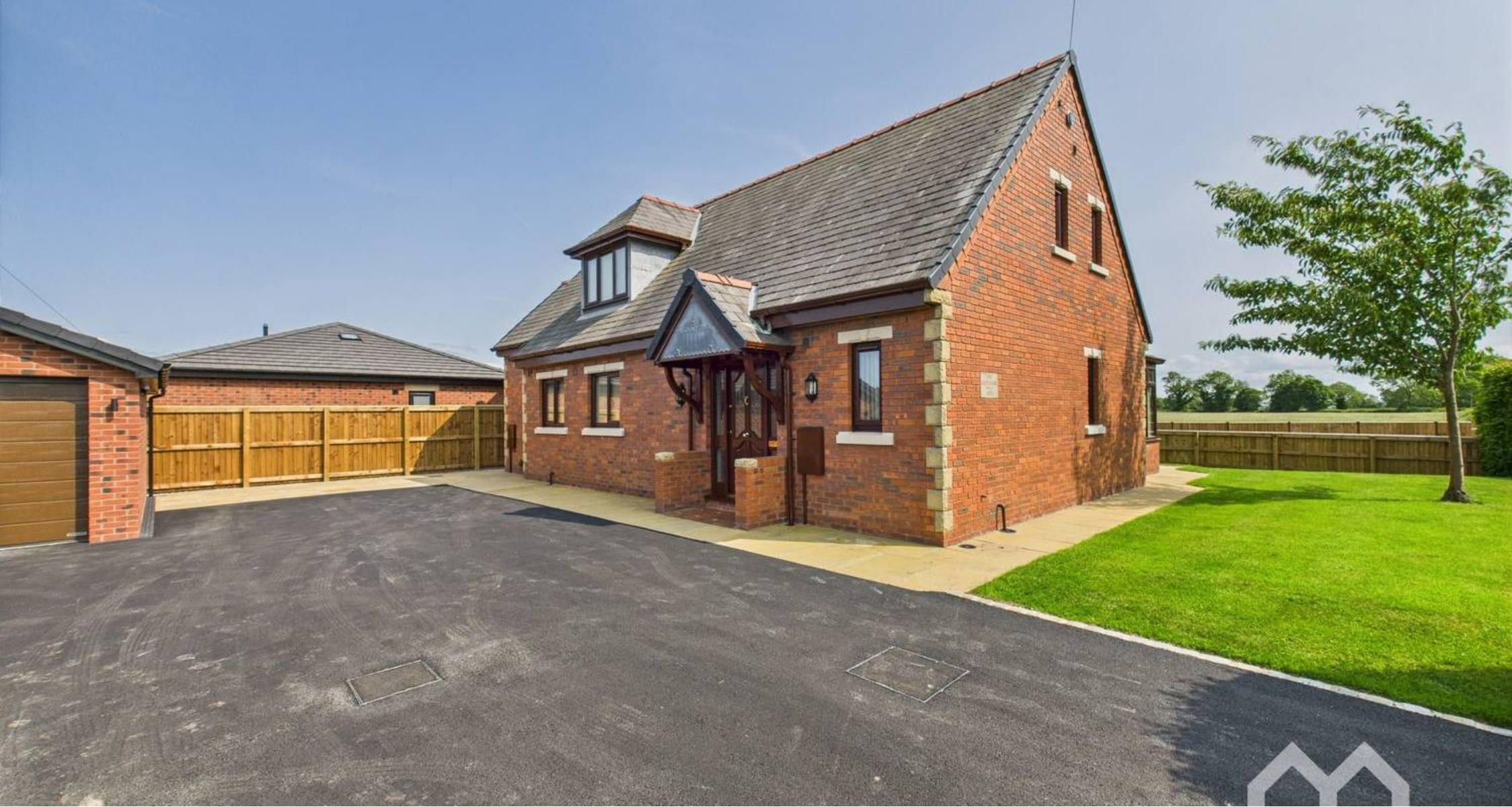
Gatehouse Nursery Lane, New Longton Preston
