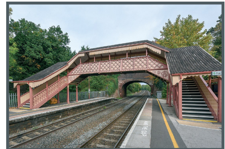
Hagley Train Station
