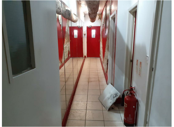
Corridor with toilet and storage room adjacent
