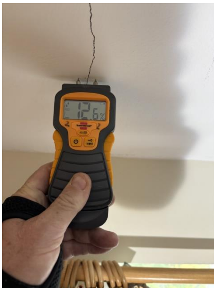
Bedroom two ceiling
