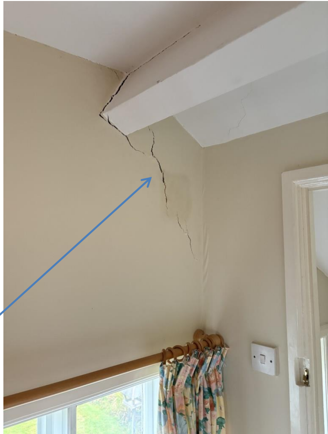
Cracked and very damp (49%) wall in bedroom 2, below the roof structural purlin.
