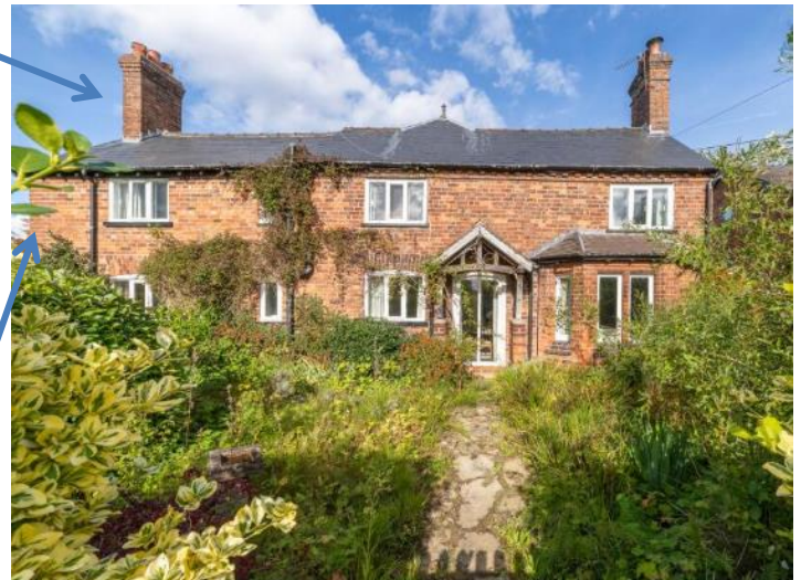
Gable end and front corner requiring underpinning
