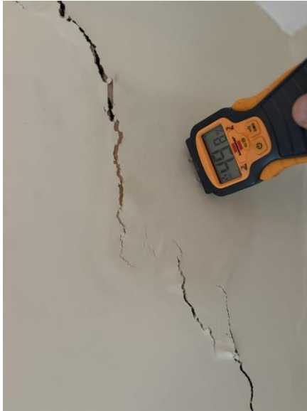
Cracked and very damp (49%) wall in bedroom 2, below the roof structural purlin.
