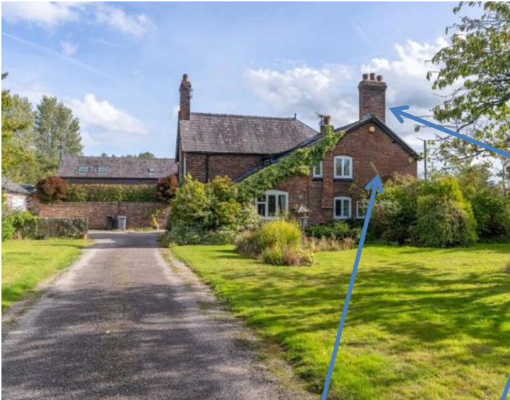
Gable end and front corner requiring underpinning
