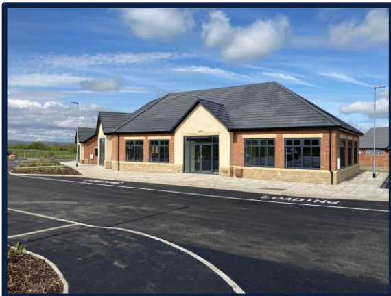
Newly constructed units
