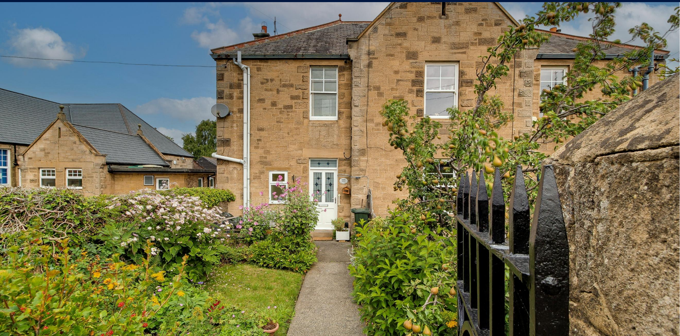
SCHOOL HOUSE, MAIN ROAD, STOCKSFIELD NORTHUMBERLAND, NE43 7NN
