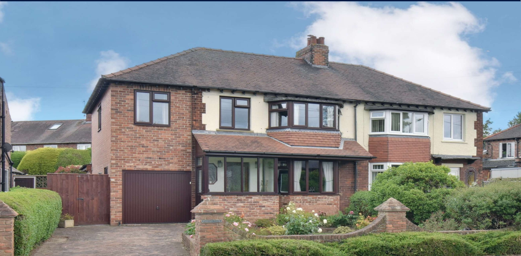
BRECKON HOUSE, 123A NORTHALLERTON ROAD, BROMPTON NORTHALLERTON, DL6 2PY
