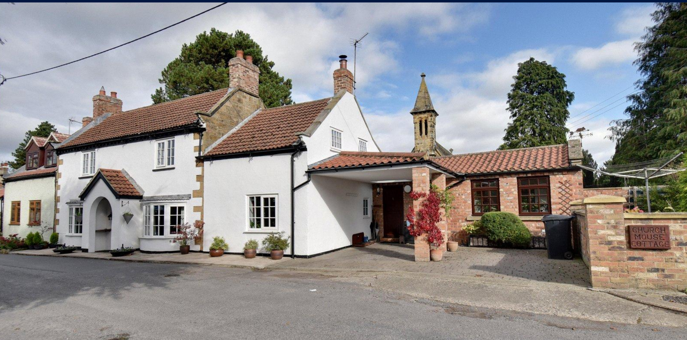
CHURCH MOUSE COTTAGE, THORNTON LE STREET, THIRSK NORTH YORKSHIRE, YO7 4DS
